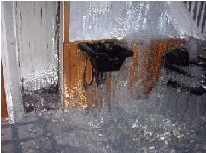
Damage can be excessive and expensive
